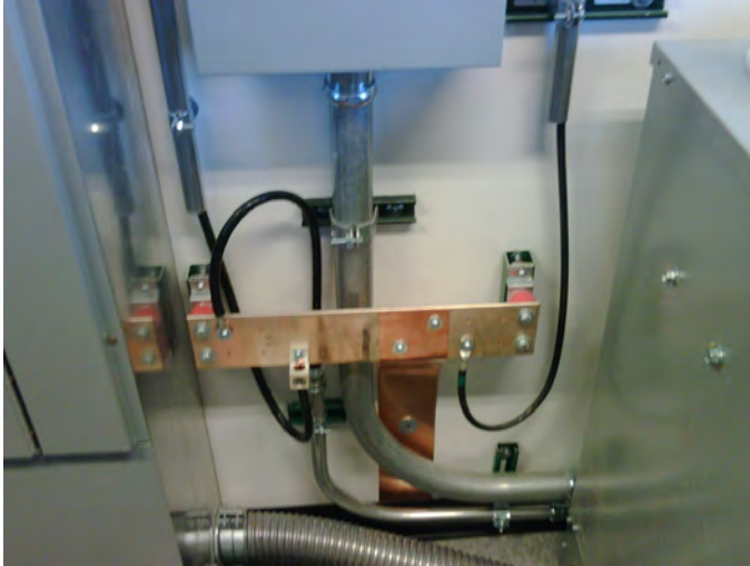
Bulkhead ground for coax cables
